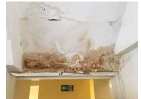
Repairs to the roof will stop water from damaging the interior of the KT building.
